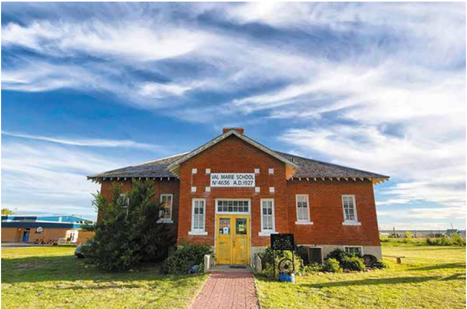
The Val Marie ecomuseum uses the old school as an interpretive centre.
